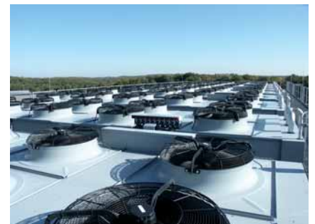
Condenser with axial fans
