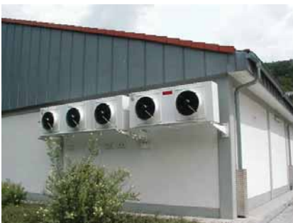
Small refrigeration units with ZIEHL-ABEGG fans
