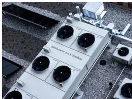
Condenser with axial fans
